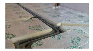
(b) Fill any voids around the pipes, with a weak sand:cement mix and level off. Then place the 2nd layer of insulation over the 1st layer, ensuring it remains flat, with no rocking.
