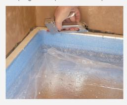
(b) Place 500 gauge plastic over the top of the insulation ensuring it is pulled tight with no creases. Overlap joints a minimum of 100mm and tape joints. Tape the 500 gauge membrane to the plastic skirt of the edging strip.
