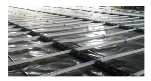
(b) Fill the underfloor heating pipes with water.
