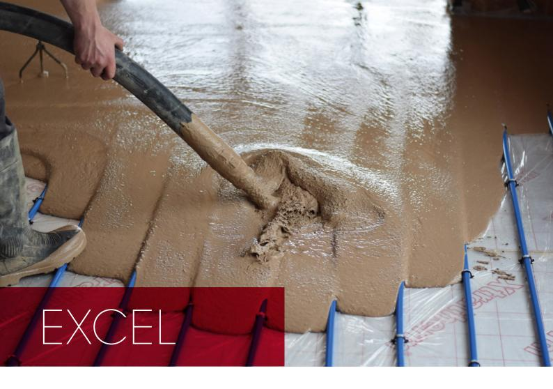
Ultraflo® is a unique hemihydrate calcium sulphate liquid floor screed designed to be used with underfloor heating. The product reduces the risk of cracking, improves heat responsiveness and heat lag with underfloor heating.
