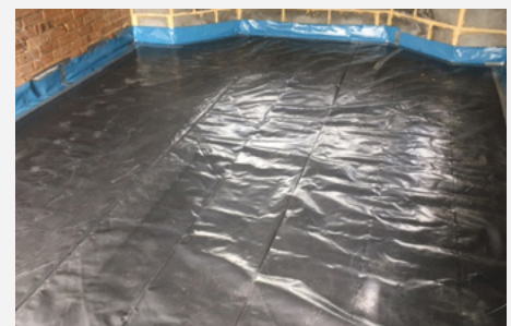
Plastic membrane laid and taped
