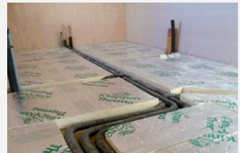
Insulation being laid
