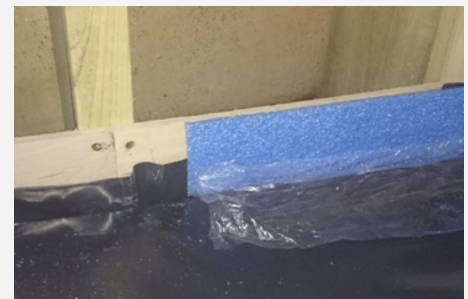
Edging strip being attached
