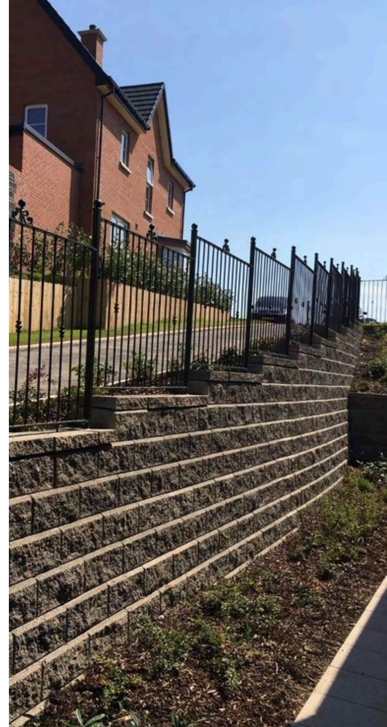
Allan Block Retaining Wall by Colinwell
